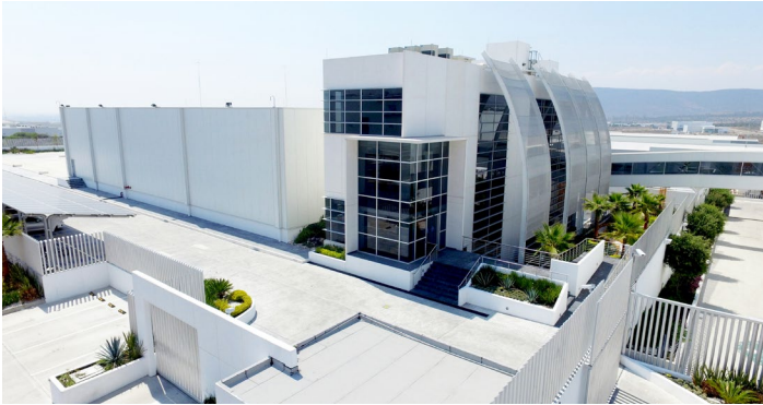
Equinix MX2 IBX data center exterior
